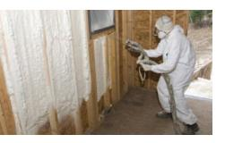
Spray Polyurethane Foam (SPF) is an insulation product that is spray-applied in situ at a building site. Two liquid components, MDI (A) and polyol blend (B) are mixed under pressure and sprayed onto a roof or wall cavity. The reacting liquids expand and solidify into a foam matrix creating a seamless seal. SPF adheres well to the area it is applied to, providing an air barrier that prevents thermal leaks.
